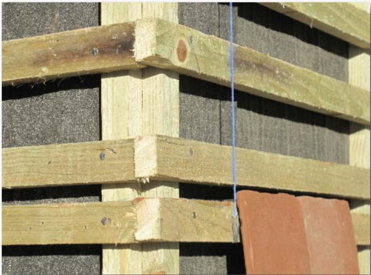
**Step 5** Starting at the right hand eaves, lay out the first row of full tiles and repeat at the top edge abutment with the soffit, and using a chalk line ping vertical lines up the battens to coincide with the side of every 5th tile. To achieve a vertical line the eaves or top course may need to be adjusted.
