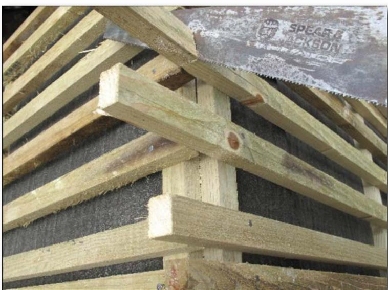
**Step 3** At the first external corner the 38mm x 25mm battens running up to the corner should be left long, and the adjacent batten running away from the corner should be butted up to the batten that has been left long, levelled and fixed into position. The excess batten should be cut off flush with the face of the batten on the adjacent wall face to produce a neat square corner ( no gaps).
