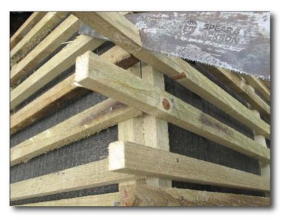
**Step 3** At the first external corner the 38mm x 25mm battens running up to the corner should be left long, and the adjacent batten running away from the corner should be butted up to the batten that has been left long, levelled and fixed into position. The excess batten should be cut off flush with the face of the batten on the adjacent wall face to produce a neat square corner ( no gaps).
