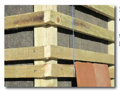
**Step 5** Starting at the right hand eaves, lay out the first row of full tiles and repeat at the top edge abutment with the soffit, and using a chalk line ping vertical lines up the battens tocoincide with the side of every 5th tile. To achieve a vertical line the eaves or top course may need to be adjusted.
