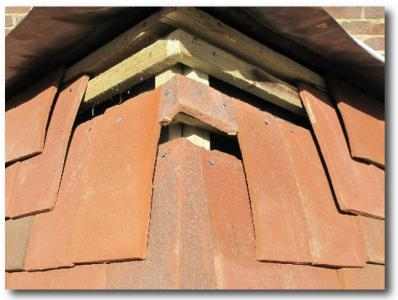
**Step 11** If in the course of the work an external angle tile is broken, and needs to be replaced. The tiles above in a large V must be stripped down to the broken tile, the broken external angle replaced and the tiles reinstalled and fully nailed back up to the top edge or gable. The use of mastic, or home made wire or metal contraptions to hold the replacement external angle tile in position, will not be acceptable.
